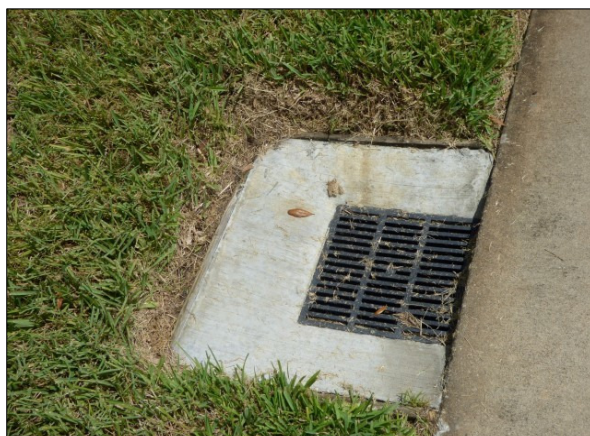
Stormwater Drainage Yard Drain
