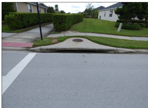
Stormwater Drainage Curb Inlet
