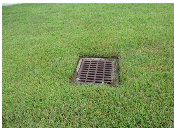
Stormwater Drainage Yard Grate Inlet
