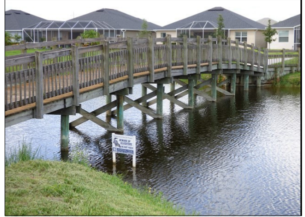
Typical Pedestrian Bridge Frame
